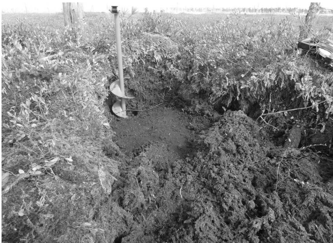
Figure 1. Conducting works to determine the thickness of frost penetration (35 cm).
