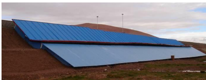
Fig.4 the QTR awning embankment
