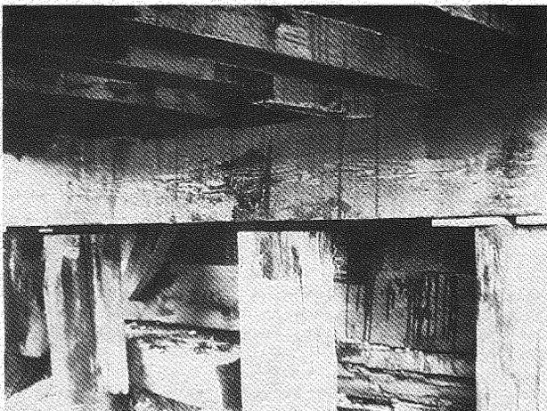
Figure 11 Gaps and shims on top of timber piles
