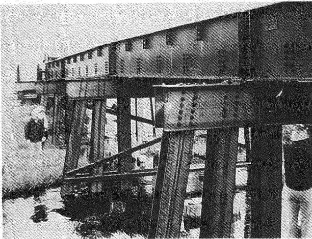
Figure 13 Steel replacement structure for Km 715 showing heave of the centre pile bent
