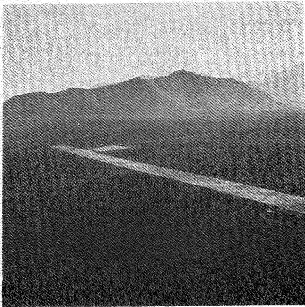
Fig. 6 Rock fill runway at Killik well site with deep fill on north end, in foreground, 1980.
