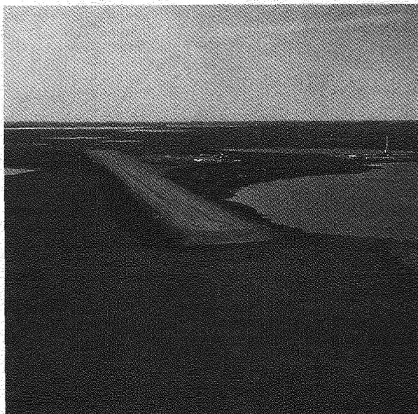
Fig. 5 Insulated runway at Inigok on sandy ridge constructed with limited gravel from Colville River, 1978.
