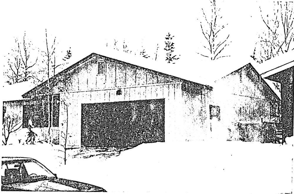
PHOTO #1: FRONT OF GARAGE AND SOUTHEAST END OF HOUSE. NOTE ELEVATION ABOVE STREET.
