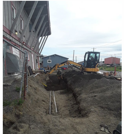
Quinhagak community members and ANTHC installing the flat-loop evaporator thermosyphons.
