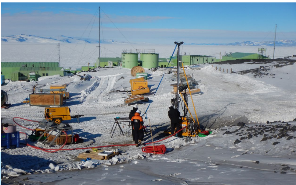
Geotechnical investigations to support the Scott Base redevelopment (2019).
