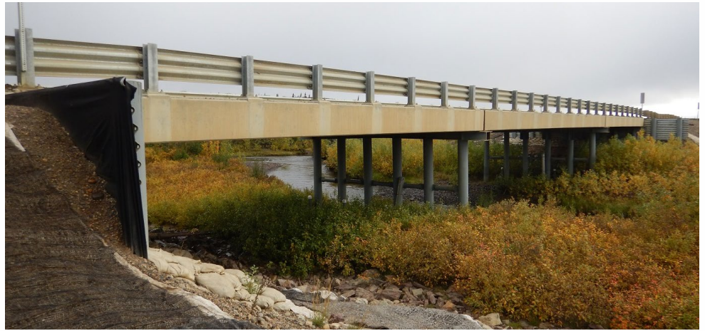
Hans Creek Bridge (ITH km 57.3).
