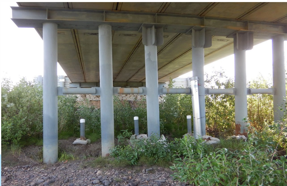
Ground temperature cables cased in white capped PVC pipe below Hans Creek Bridge.
