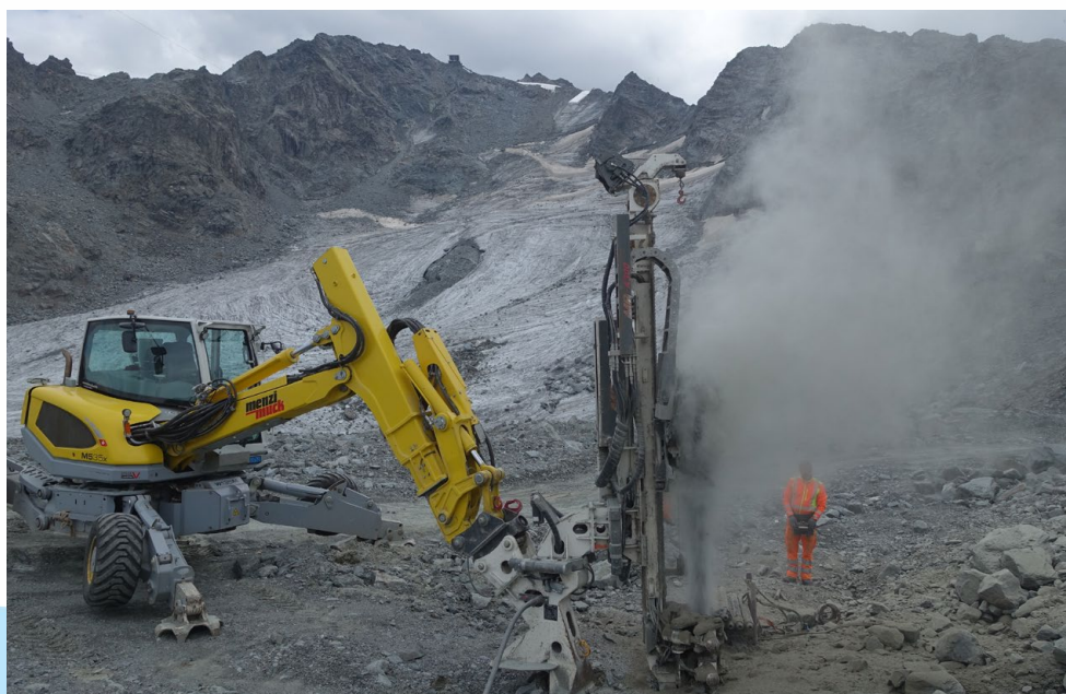
Borehole replacement at the Gentianes PERMOS Site, Swiss Alps (summer 2022) by UNIL to ensure the continuation of the 20-year temperature time series. Photo: Christophe Lambiel.
