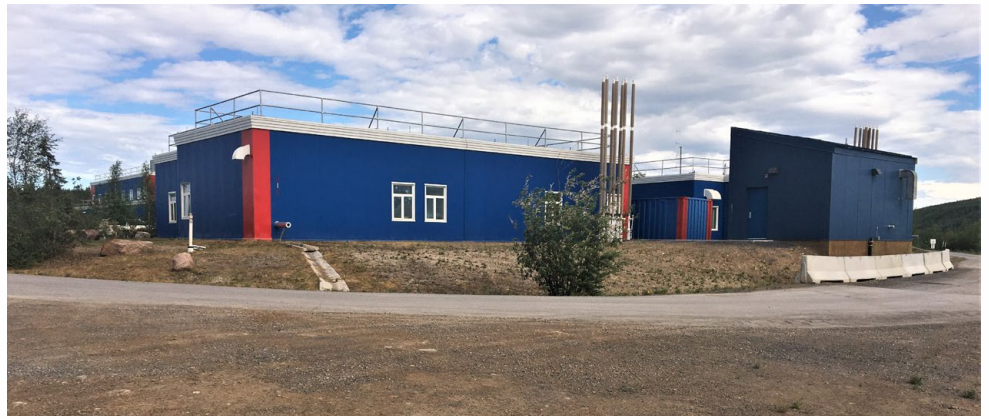
North facing view of the Inuvik Regional Hospital, NT, with flat-loop thermosyphon system.
