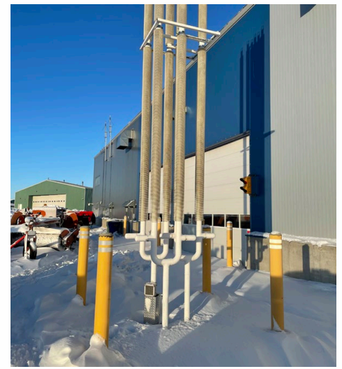
A radiator bank with a D405 Data Logger installed near the base.
