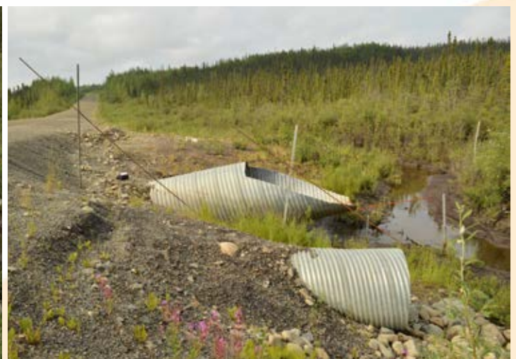
Fig. 2. Left: new culvert installed at YT km 32, Dempster Highway in the North Klondike River Valley after failure of the infrastructure due to ice blockage in 2014. Photo taken in 2017. Right: failure of the culvert due to icing development two years later (2019).
