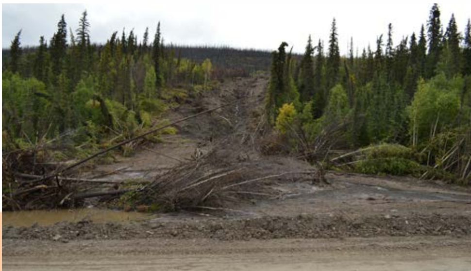
Fig. 4. Landslide that blocked the Dempster Highway at YT km 243 following heavy rain (2018).
