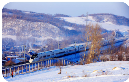
A high speed train operating in winter on the Harbin to Dalian railway.
