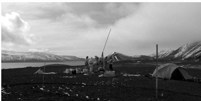
Drilling permafrost monitoring boreholes at the Crater Lake CALM-S site, Deception Island, Antarctic. A collaboration between Argentina, Portugal, Russia and Spain in the framework of the IPY TSP project. (Photograph provided by Gonçalo Vieira)
