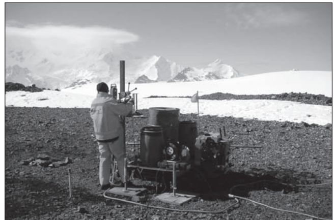
Drilling a permafrost monitoring borehole at Reina Sofia hill, Livingston Island, Antarctic. Projects PERMANTAR/PERMAMODEL. (Photograph provided by Vanessa Batista)
