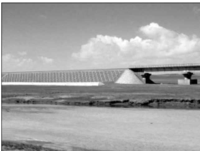
Qinghai-Tibet Railway bridge embankment. Photograph provided by Huijun Jin.
