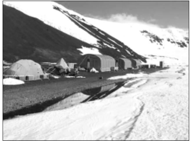
Cape Hallett Camp, January 2004. Photograph provided by Megan Balks.
