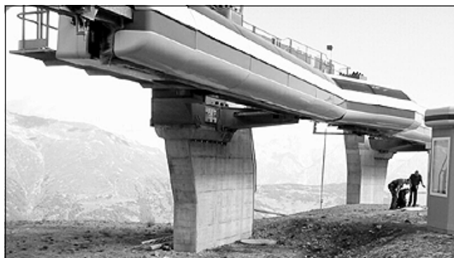
Unstable chairlift pylons in creeping permafrost terrain (Photograph courtesy of Marcia Phillips.)
