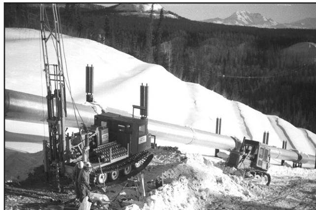
Winter drilling on permafrost slope. Photo: Bucky Tart.
