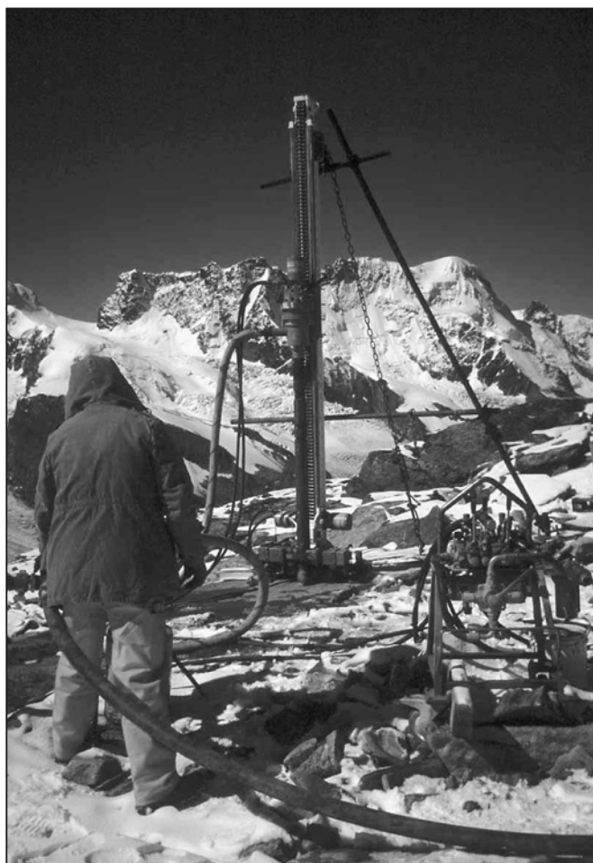
Drilling operations at Stockhornplateau. Photo: Thomas Herz
