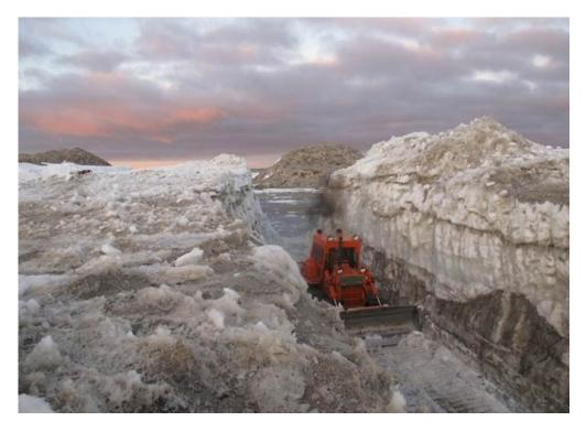
Figure 2: Image shows excavation of site to verify stratigraphy suggested via GPR.
